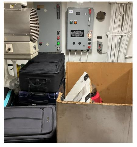
Excess equipment and storage. Note the space heater to the left within inches of cloth luggage. Everything is blocking electrical breakers. If there was an electrical fire it will not be easy to reach the breaker safely to secure power to that system. (Photo Credit: Mr. Robert Penner)
